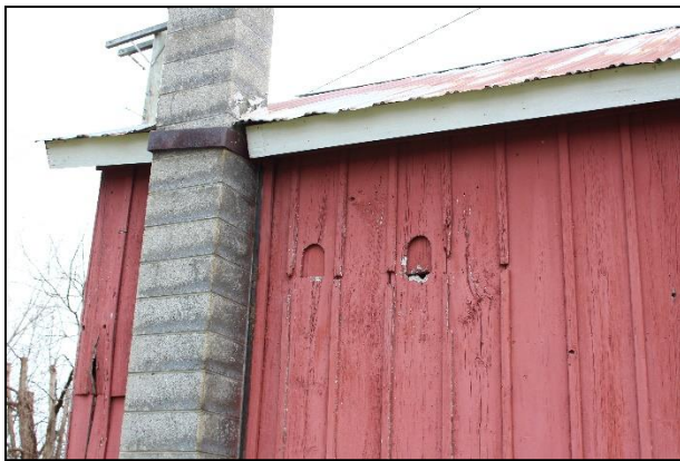
Figure 46. Chimney and patched opening on Garage, east end of north elevation.
