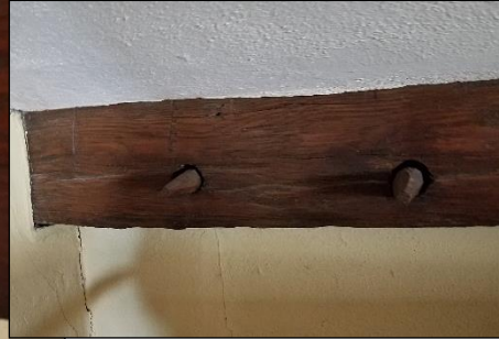
Figure 32 (left). Paired eight-sided pointed pegs along plate on west elevation of Wing.
