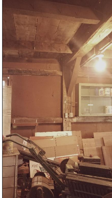
Figure 43 (left). Garage, interior view of mortise and timber joinery, southeast corner of building.
