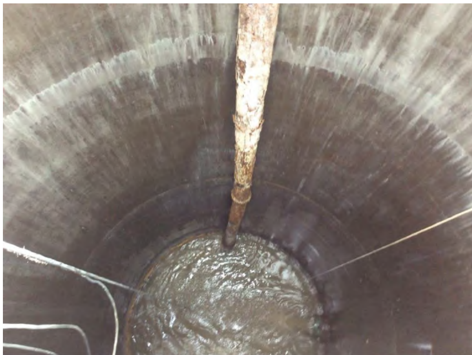
Photo 34: Wet Well Bypass Pump Line
