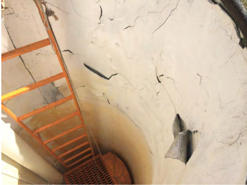
Photo 10: Steel Can Interior Coating System
