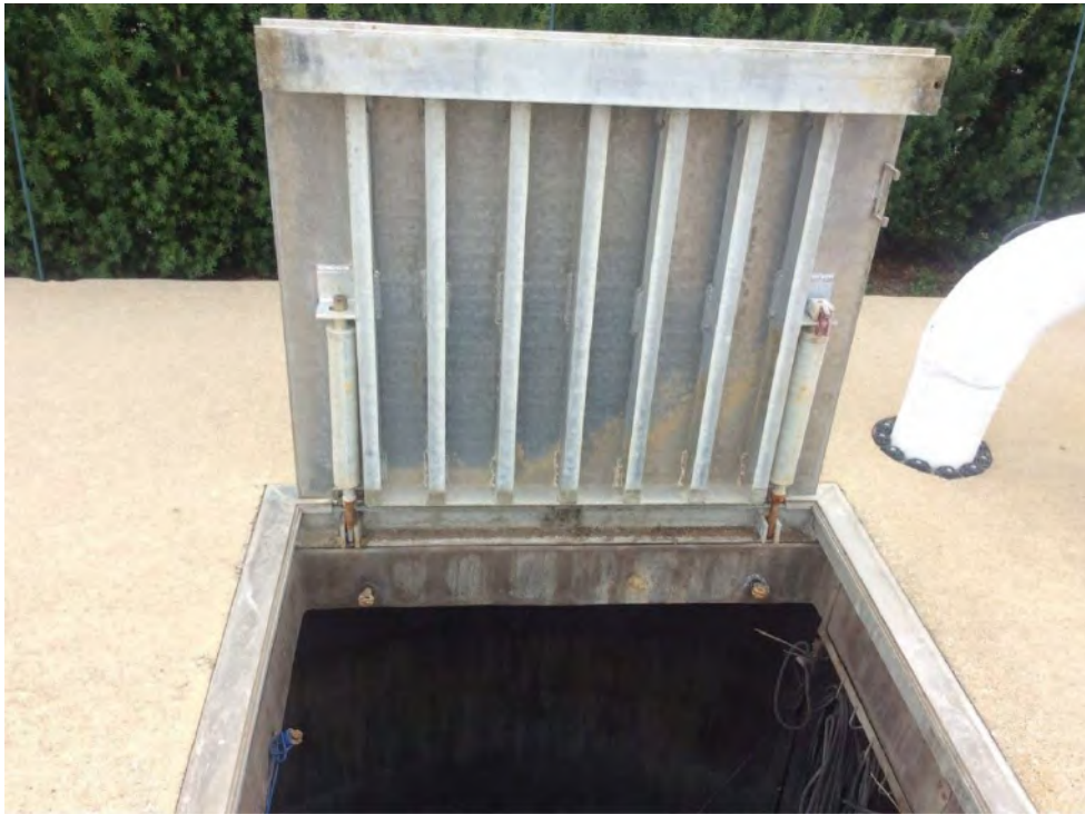
Photo 35: Wet Well Access Hatch
