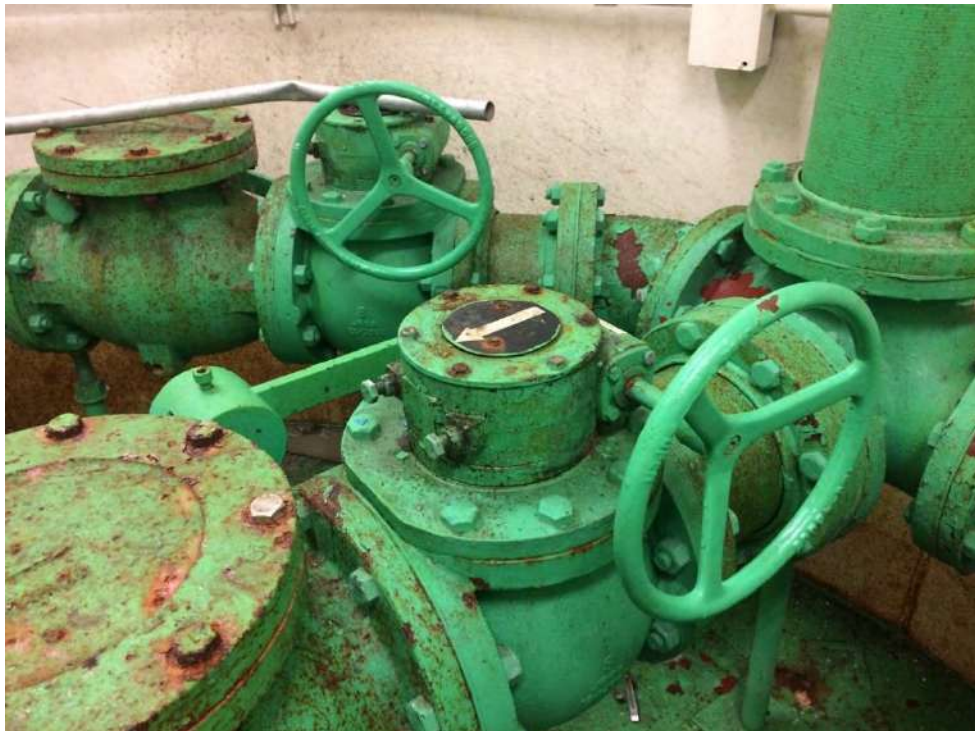
Photo 4: Forcemain Piping Paint System
