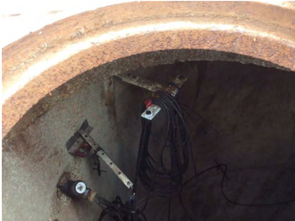
Photo 21: Wet Well Float Rack
