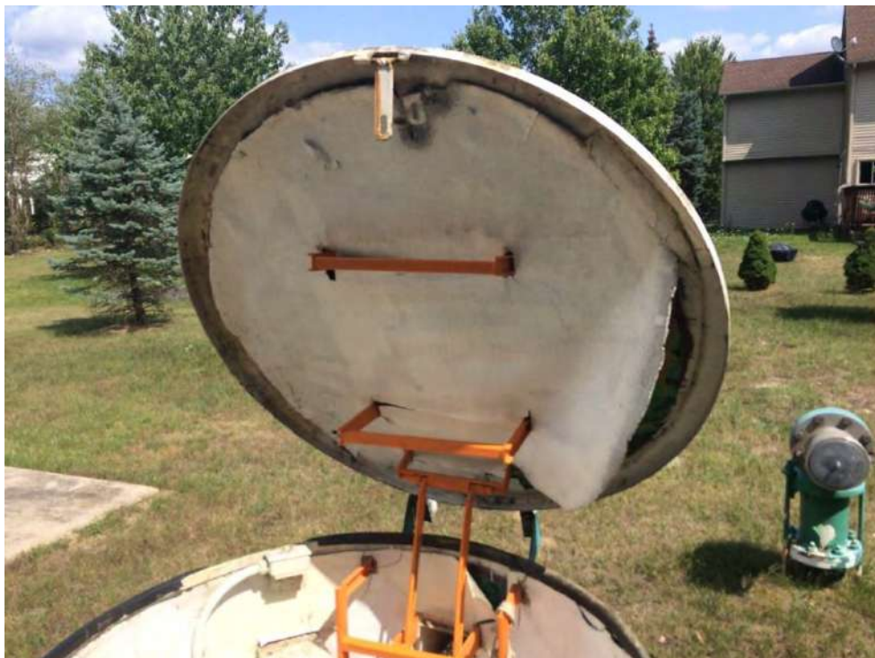
Photo 9: Steel Can Access Hatch
