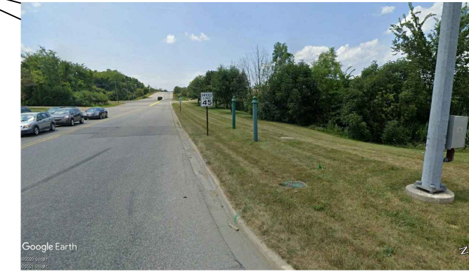
Carpenter Road and Ellsworth Road (Lowe's Looking West)
